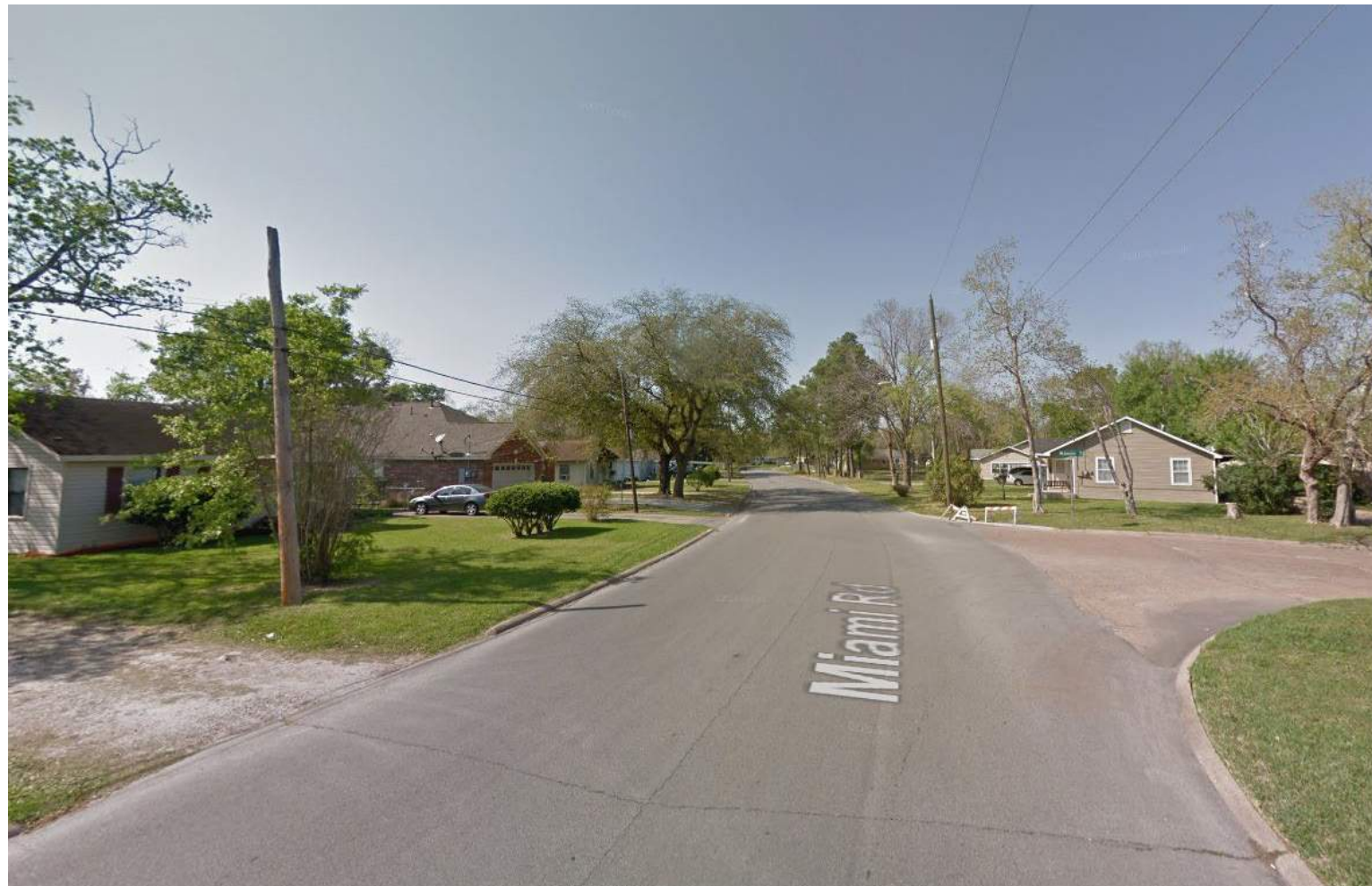
Existing Condition - Miami Dr looking north
