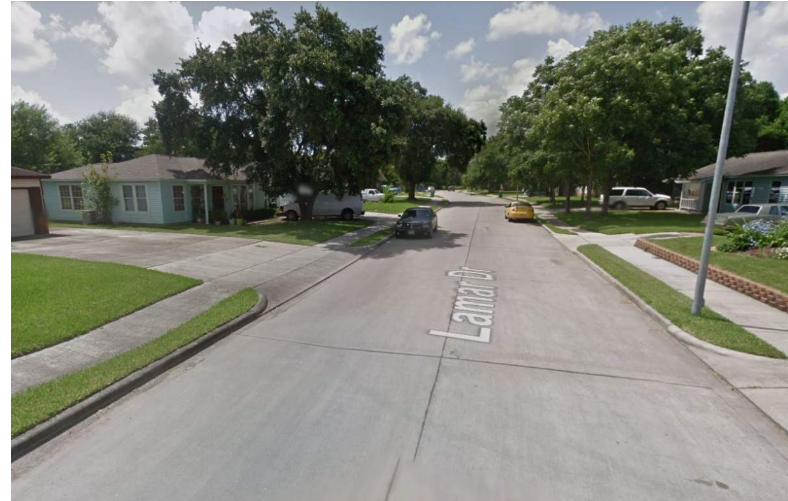
Existing Condition - Lamar Dr looking north
