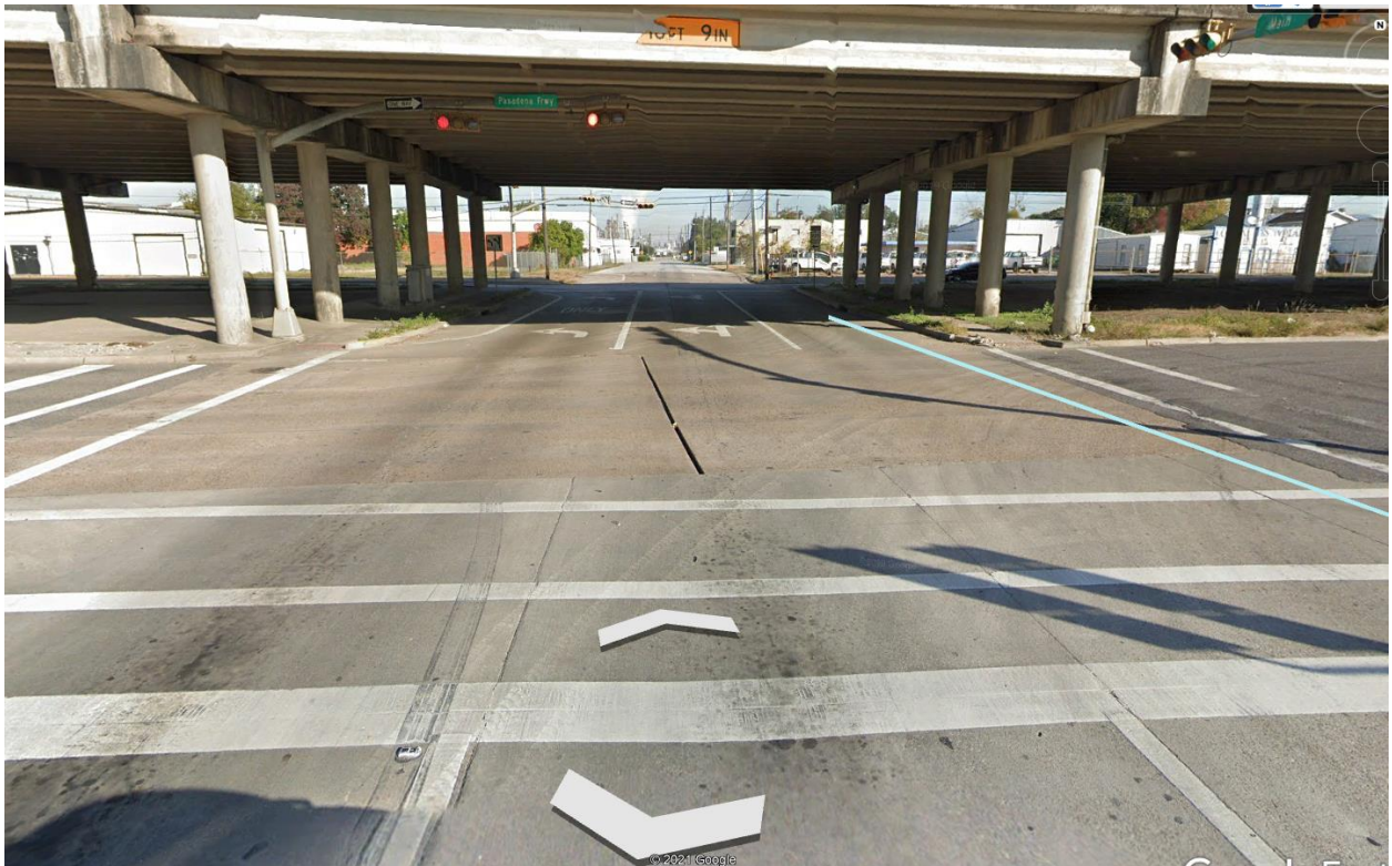
Main Street Intersection- the installation will terminate on the west side of the street before reaching the lighted intersection.
